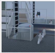
9 Check input and output valves of slave pump (open)
