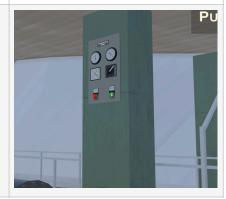
11 Start slave pump (If slave pump does LO SLAVE PUMP CONTRO not run) 12 Go front of local panel of LO Master LO MAS pump 13 Stop master pump 14 Close input and output valves of master pump 15 Repair the master pump
